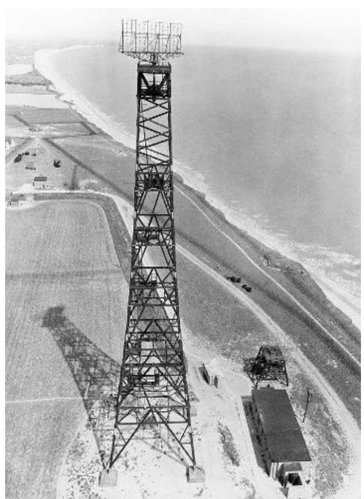
A Chain Home Radar Station at Hopton-on-Sea
